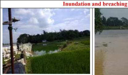
Figure 53: Ring band protection with Gunny bag at breach point (during 2017) of Damodar Right Embankment near Tokapur River Lift point
