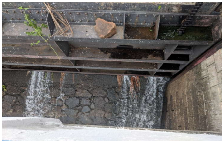
Leakage through gates of Indpur Canal Head Regulator
