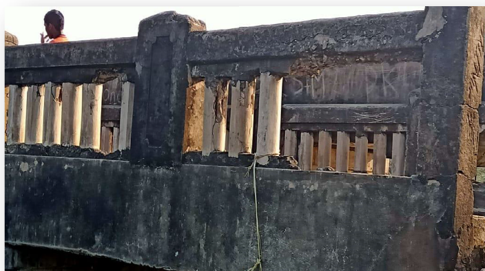
SMC tail regulator bridge parapet wall in damaged condition
